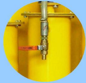
*Cooling water bypass valve for
