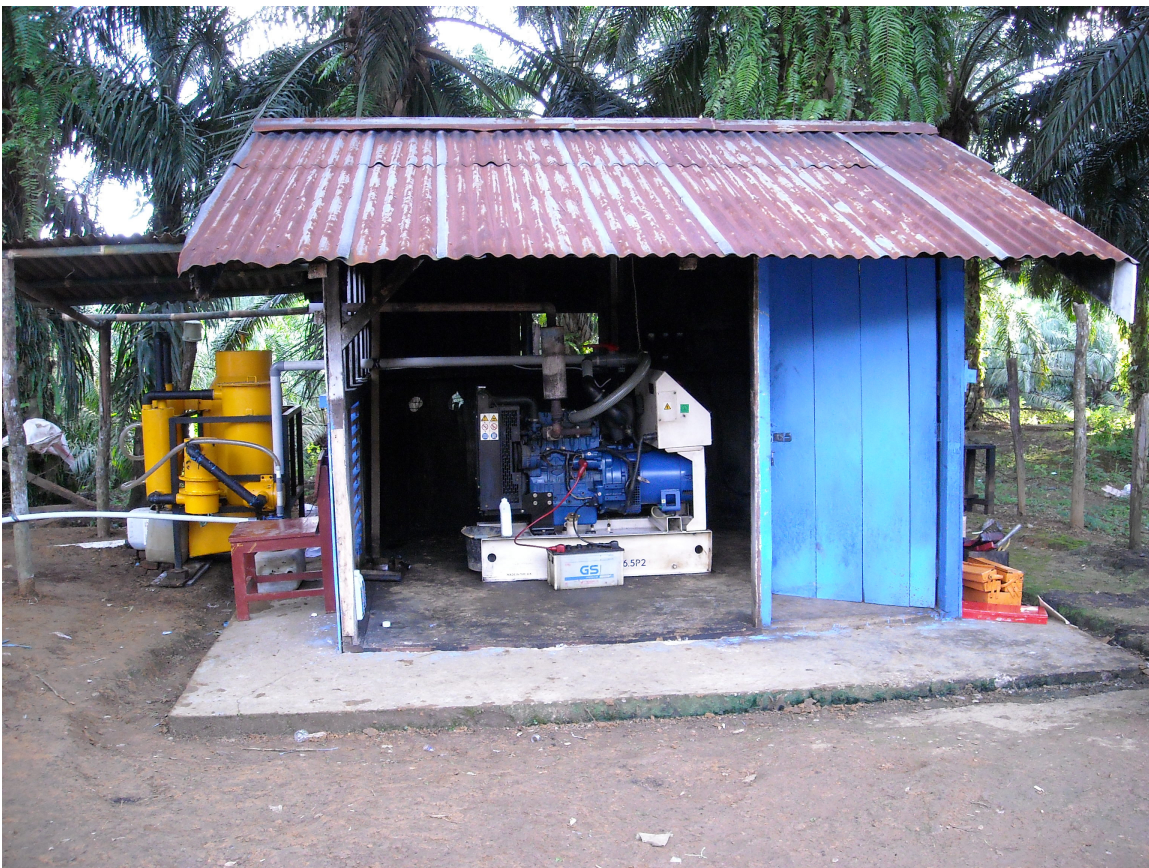
Fig 5. Model TG 30 operating in PT Daria Dharma Pratama's palm oil plantation in Ipuh, Bengkulu, Indonesia using palm oil kernel shell.
