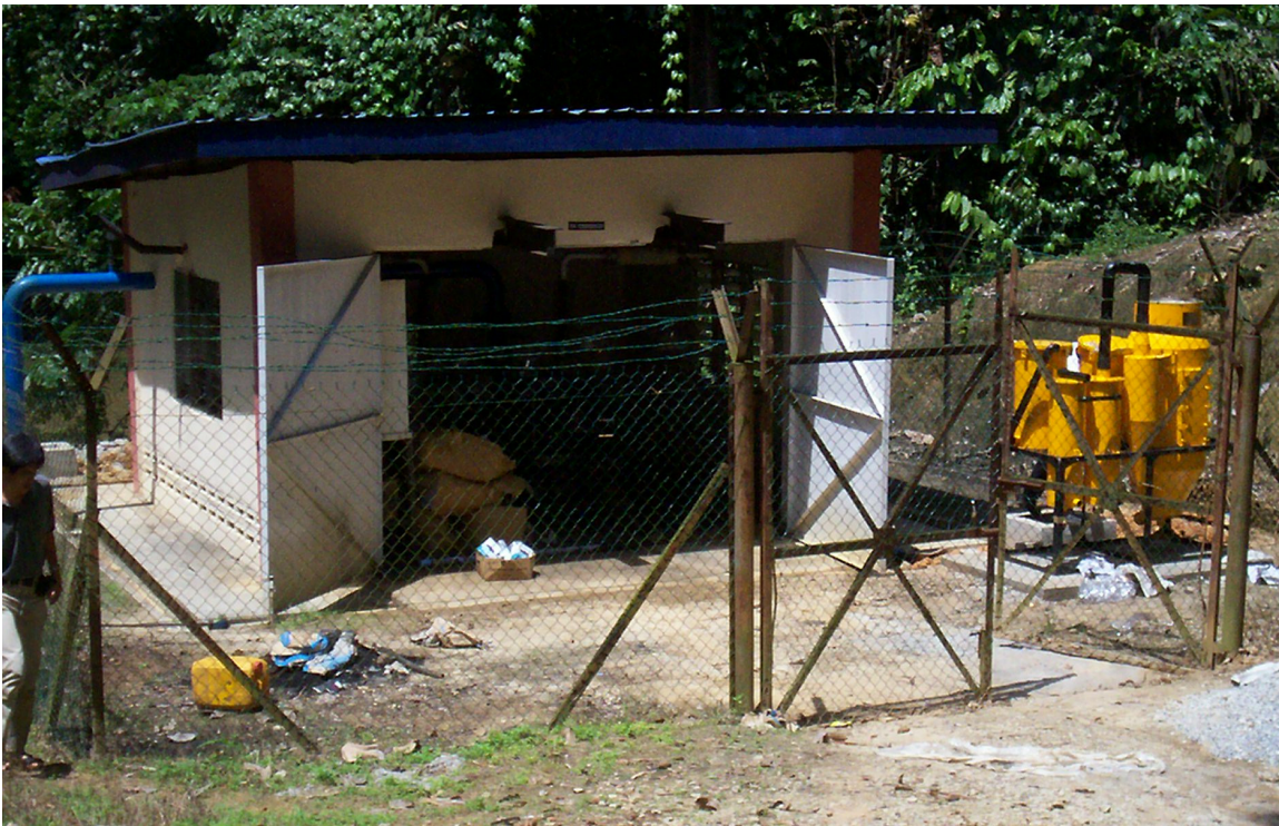
Fig 6. Model TG 70 operating in Felda Palm Industries Sdn Bhd in Kuala Lipis, Pahang, Malaysia using palm oil kernel shell. The gasifier is powering two Lister Petter engine driven water pumps supplying water to a palm oil mill 13 km from this site.
